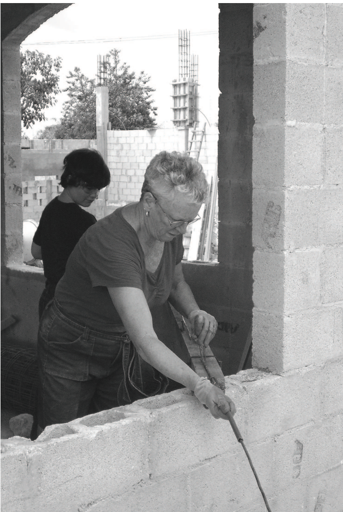
Claudia Sharpless straightens steel rebar
